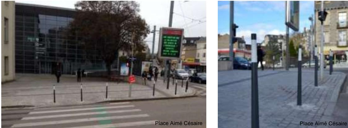
Figure 43. Ceramic bollards Photographic credit: © Ville de Limoges
