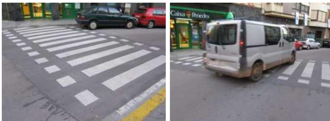
Figure 32. Ceramic tiled zebra crossing. Onda. (Source: ITC)
