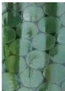
Figure 25. Porcelain shaped by extrusion and die cutting. Maritime walkway, Benidorm
