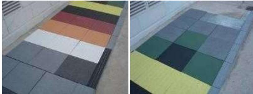
Figure 8. Haptic pieces designed with optimal reliefs for pedestrians.
